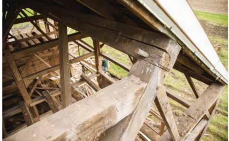
Many of the structures were built entirely by hand, which means they are held together with unique cuts and joints. This contributes to the time it takes to bring down a building and heightens the importance of the notes taken on the building during that process.
